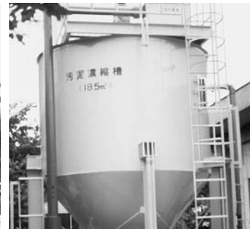
攪拌式汚泥濃縮槽 Agitation Type Mud Condensation Tub 口径・・・φ3200×高3800 減速比1/2537、 Caliber: 0.75kW-4P φ3200×Height3800 Reduction ratio 1/2537 0.75 KW-4P
